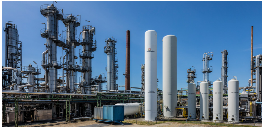
From production sites to technology parks with various production processes
